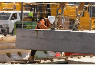
The scope of works included staged demolition of Wharf 1 and 2's existing relieving slabs, fabrication, transportation and placement of 110 precast panels at 7m x 3m and weighing 30t, as well as the decommissioning and recommissioning of under deck services.
