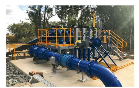
Pensar designed a custom hose reeling machine and pump catch tray to enable the pumps to be pulled from the depths of the river and be maintained without having to be disconnected from the flexible rising main.
