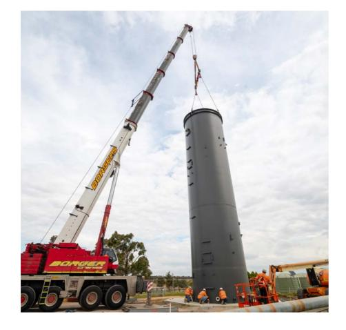
The existing Minimbah potable water storage tank required an upgrade along with the addition of a newly constructed standalone steel circular reservoir.
