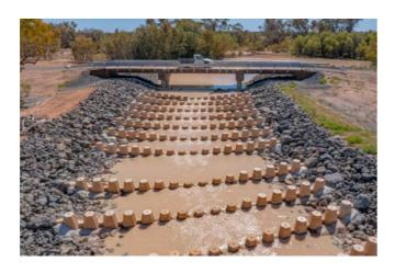
Pensar also completed the temporary works design. Pensar successfully installed the Homestead Dam Bridge using an InQuik bridging system in 21 days from foundations to completion.
