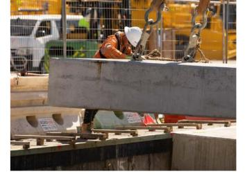
fabrication, transportation and placement of 110 precast panels at 7m x 3m and weighing 30t, as well as the decommissioning and recommissioning of under deck services.
