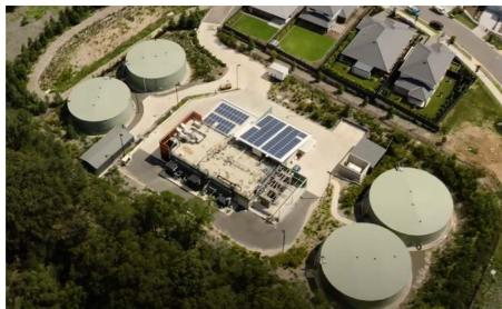
This two-stage project involved the construction of a new greenfield local water centre via an MBR plant to service the new subdivision.
